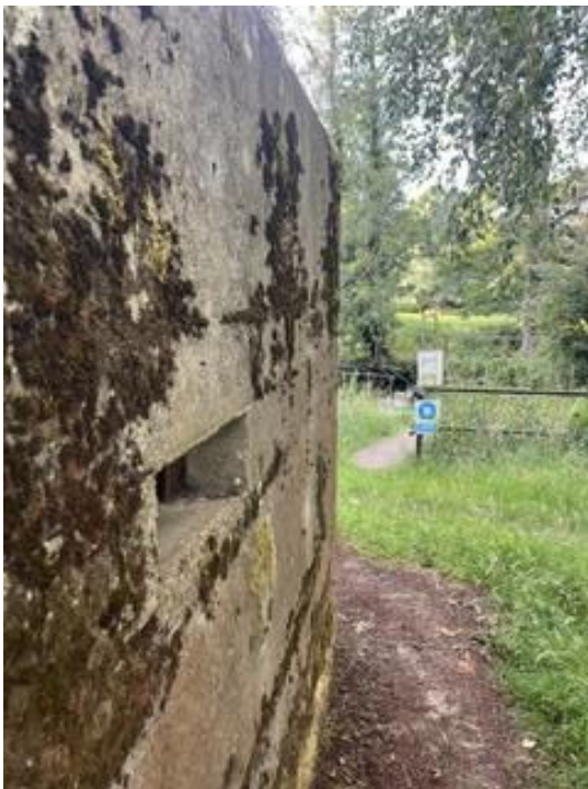
WW2 Pill Box at edge of River Colne
